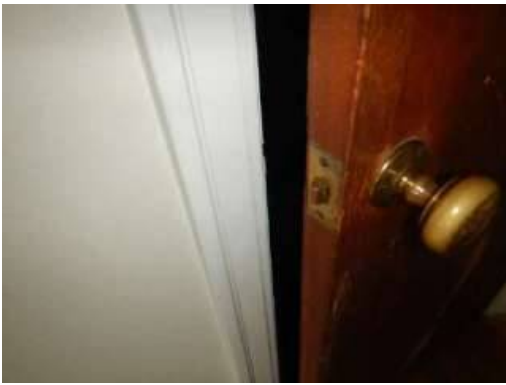
Photo 31-9 @ attic back bedroom & closet
