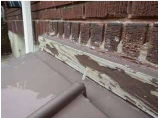
Photo 4-3 @ lintel over hatch
