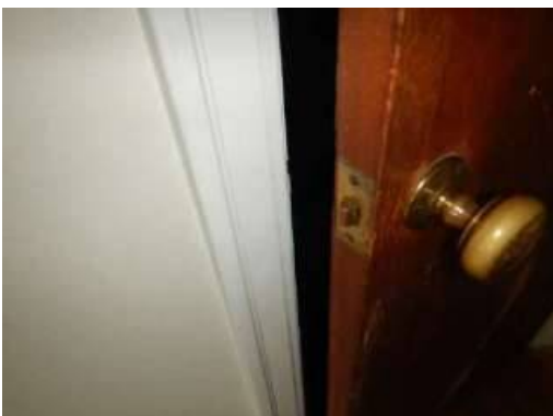
Photo 31-9 @ attic back bedroom & closet
